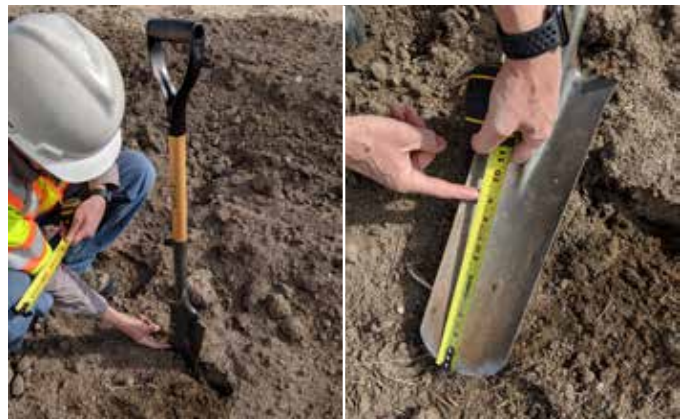
Photo 5. Depth of topsoil placement verification in the field.
