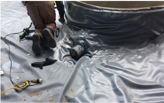
Photograph PPS-19. Underdrain penetration of geomembrane with boot. Photo: Creative Civil.
