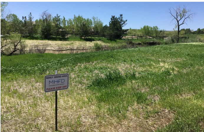
Photograph RPA-5. Grass buffers are well suited for use in riparian zones to assist in stabilizing channel banks adjacent to major drainageways and receiving waters.
