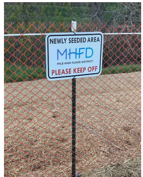
Photograph RPA-11. Signage and construction fencing can help protect the RPA as vegetation becomes established.
