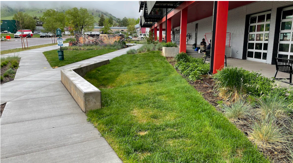
Photograph RPA-9. Grass buffer provides an opportunity for filtration and infiltration of roof runoff and disconnects impervious area of roof from inlet to storm drainage system.
