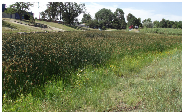
Photograph RP/CWP-8. Barnum Park constructed wetland park shows transition from hydrophytic rushes to upland grasses.
