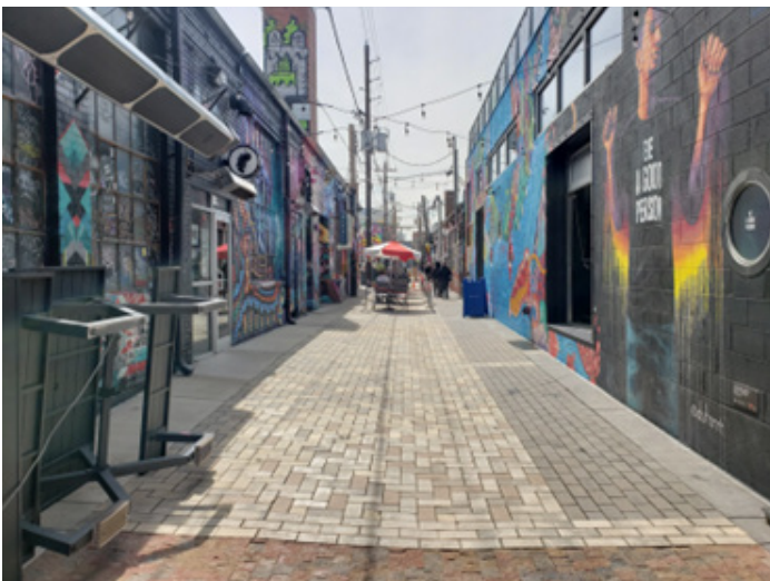
Photograph 4-1. Permeable pavement in an alleyway provides filtration in a space-constrained environment and provides a multi-functional area valued for more than just stormwater treatment.
