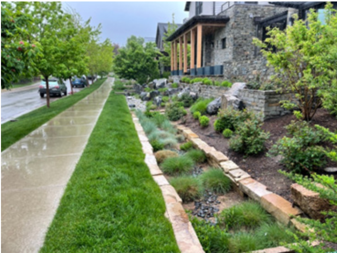
Photograph 4-3. Choice of materials for bioretention system is compatible with landscaping and aesthetics of neighborhood.
