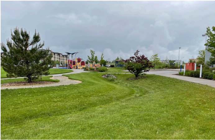
Photograph RPA-3. This grass swale provides treatment of runoff from a parking lot, portions of the building, and sidewalks at a healthcare facility. Photo: WWE.
