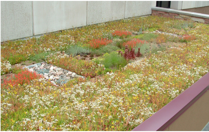
Photograph GR-1. Extensive Green Roof. Photo: Jennifer Bousselet.
