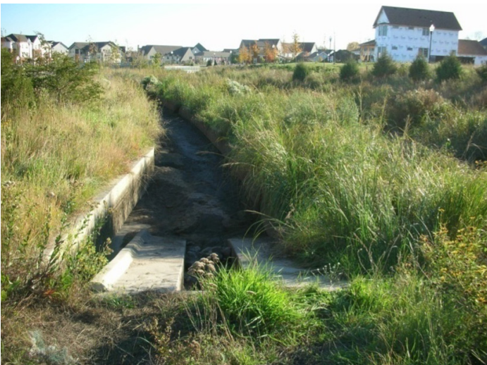
Photograph 4-11. Concrete ramp provides maintenance access to blind swale. Photo: Wenk.
