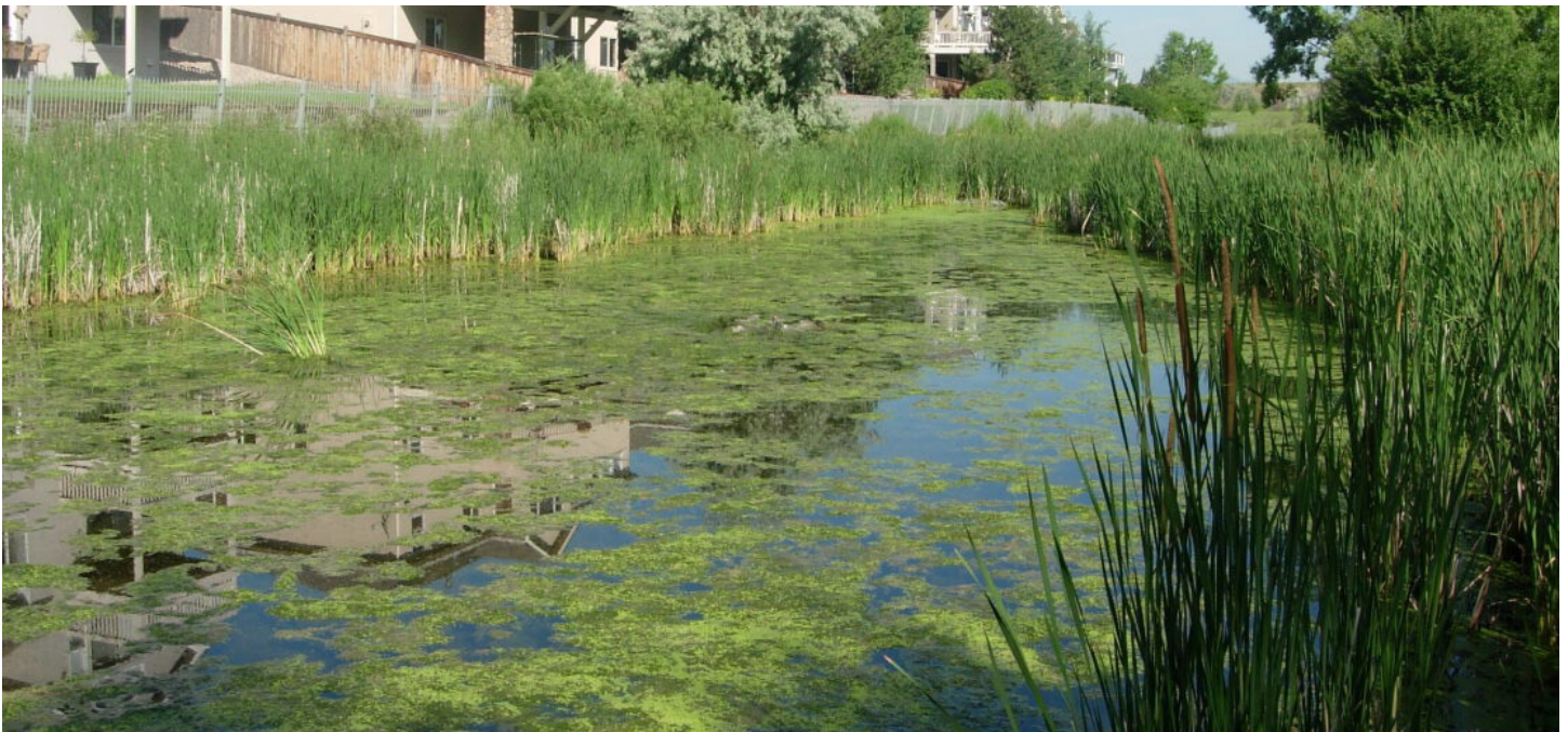
Photograph RP/CWP-6. Exceeding the minimum requirements for the permanent pool volume and depth can help to mitigate excessive growth of algae. Source control measures in the watershed that reduce nutrient loading may also be necessary.
