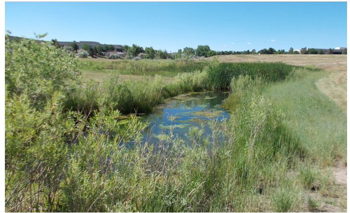
Photograph RP/CWP-2. Constructed wetland pond with diverse vegetation provides sedimentation, filtering and biological treatment.
