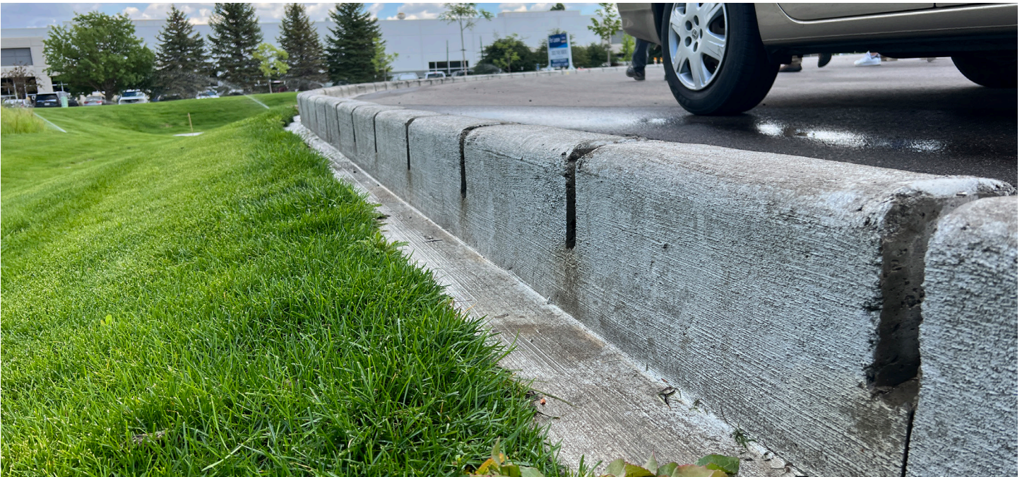
Photograph 4-8. Typical slotted curb showing drop from slot to adjacent pervious area to allow for growth of vegetation and sediment accumulation. This area provides for mowing and maintenance access to keep positive drainage from the parking lot to the RPA.
