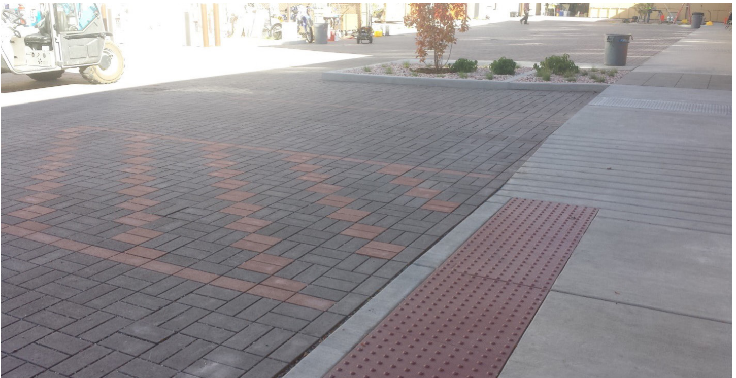
Photograph PPS-8. PICP with striped ADA parking and tree planter. Photo: Creative Civil.
