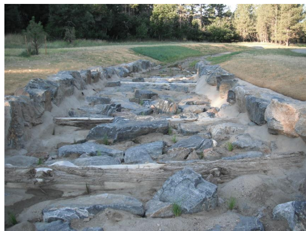
Figure 4: Post Flood Repairs
