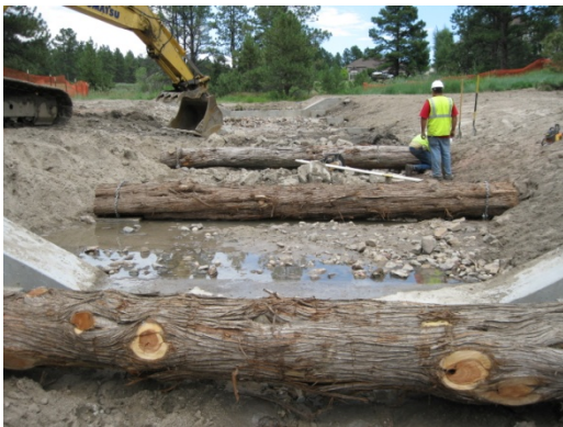
Photo 13: Install Next Log
