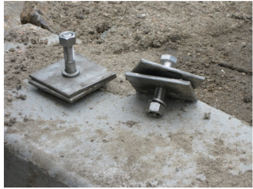
Photo 10: Prepare Anchoring Hardware
