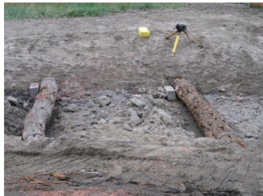
Photo 14: Finish Grading and Place Riprap
