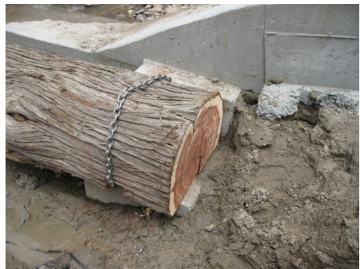
Photo 12: Finished Log on Anchor with Chain
