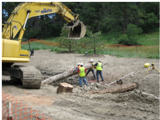
Photo 8: Place Log on Concrete Anchors
