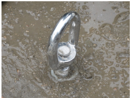
Photo 6: Place Embeds in Wet Concrete
