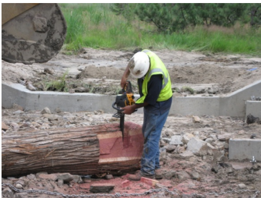
Photo 7: Notch Log for Level Crest
