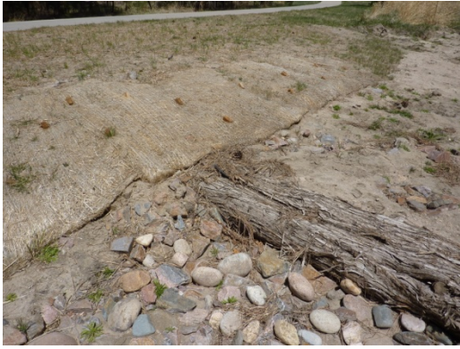
Photo 15: Install Seed and Erosion Control
