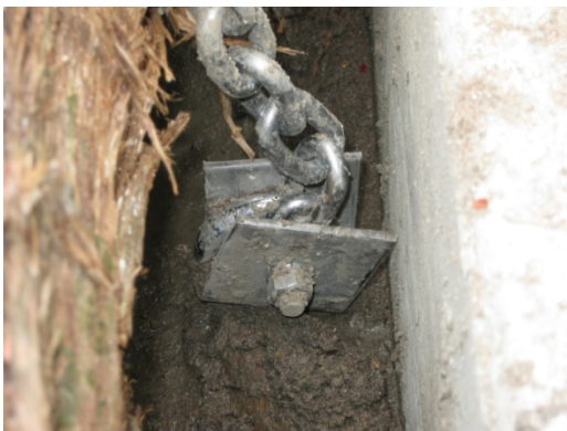
Photo 11: Attach Chain to Eye Bolt
