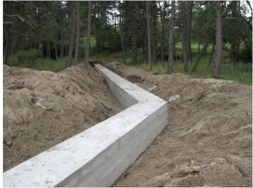
Photo 4: Place Concrete Cap
