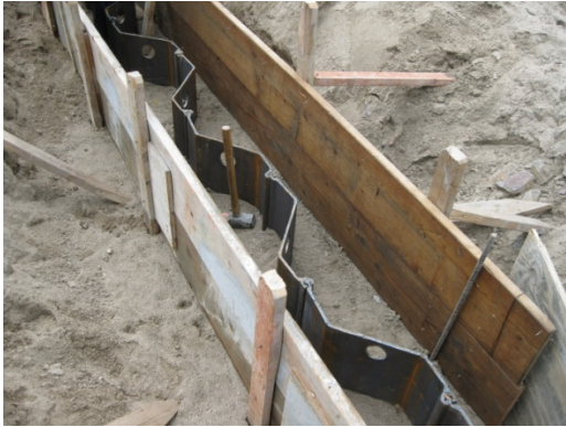
Photo 3: Place Sheet Pile and Form Cap
