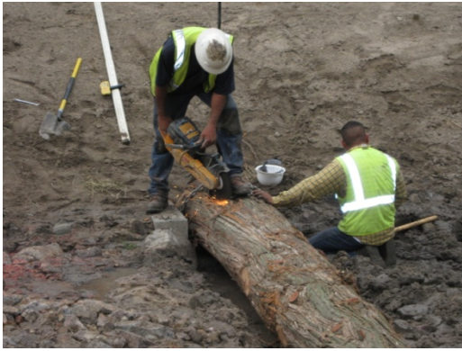
Photo 9: Cut Anchor Chain to Length
