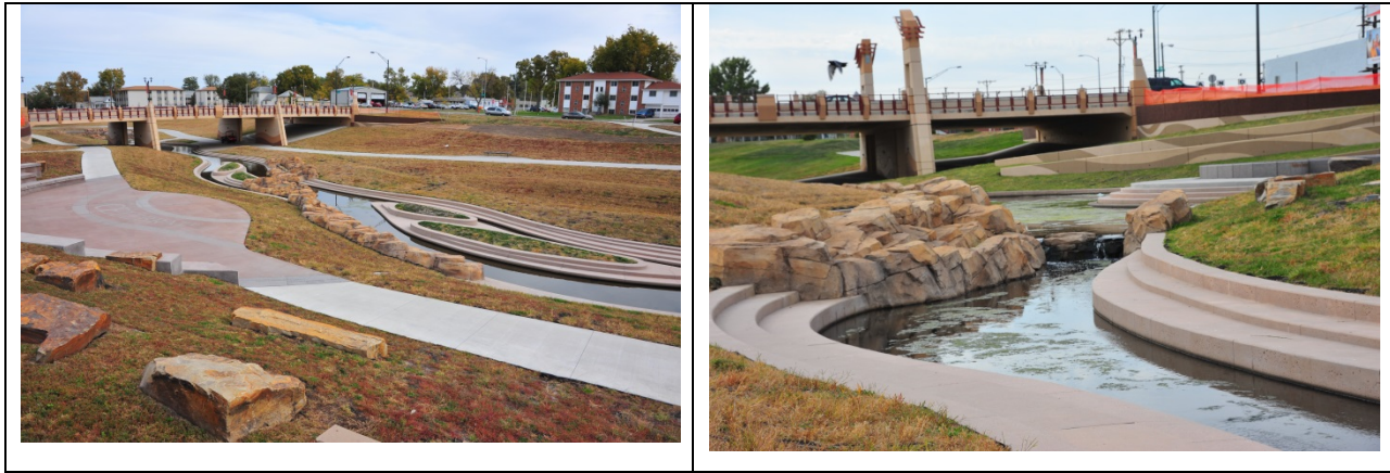
Antelope Creek near downtown, Lincoln, NE, showing paths and small amphitheatres as part of flood-proofing reconstruction projects. (Photos courtesy Bob Pitt.)
