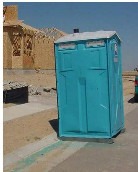
Improperly placed portable toilet with biocide running down gutter toward storm drain. (Photo courtesy of Wright Water Engineers.)
