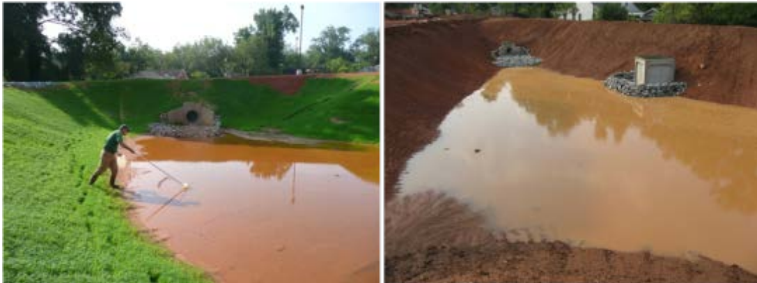
Photos of Construction Sediment Basin in South Carolina Study, after and prior to vegetation, respectively. Photos courtesy of John Hayes and Calvin Sawyer.
