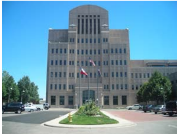
Photograph 2. Denver Public Works Building (Left of island: porous asphalt, right of island: PICP).
