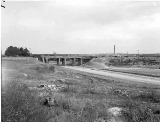
Construction of I-25 (1948)
