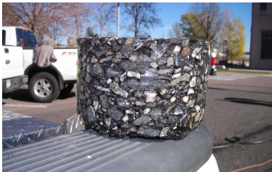
Photograph 3. Porous asphalt wearing course. Core taken in 2011.
