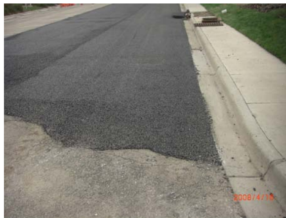
Photograph 1. The porous asphalt site with sampling inlet shown in the background
