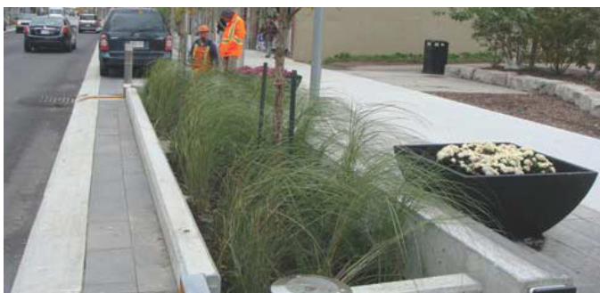
FIGURE 2. Example of stormwater planter
