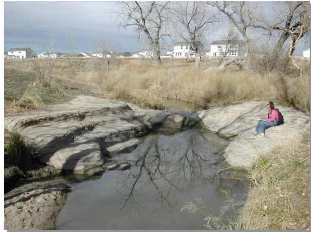
Photograph 9-8. The first sculpted concrete structure in the UDFCD region was along Grange Hall Creek in Northglenn, Colorado. The shape and color was chosen to blend into the existing landscape which consisted of native grasslands.
