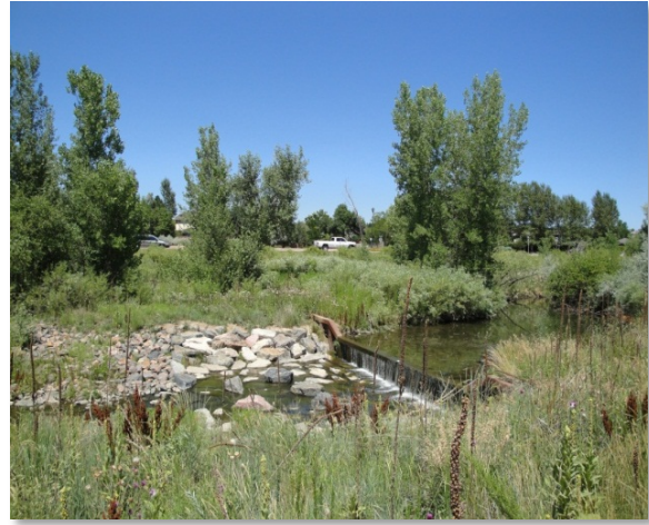
Photograph 9-27. Keeping vertical drops small improves safety during both wet and dry conditions.
