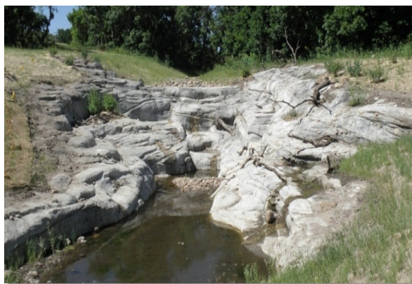
Photograph 9-10. This drop structure located along Oak Hills Tributary represents a complex design example.
