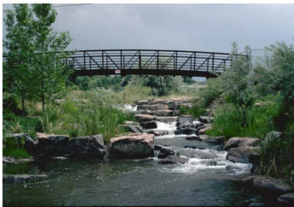
Photograph 9-1. This grouted boulder drop structure exemplifies the opportunity available for creating an attractive urban hydraulic setting for a riparian corridor.
