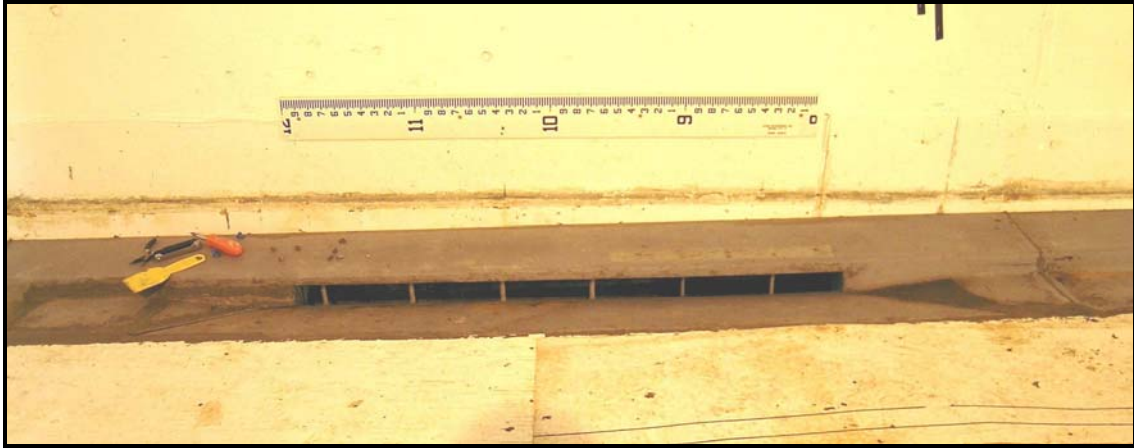
Figure 3-25: R12 curb inlet photograph
