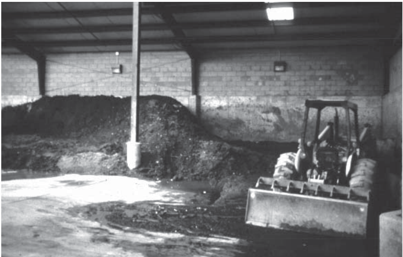
Settled vector solids at Bellevue, WA. vector decant station. Photo courtesy of Ventilation Power Equipment, Inc. , Seattle.
