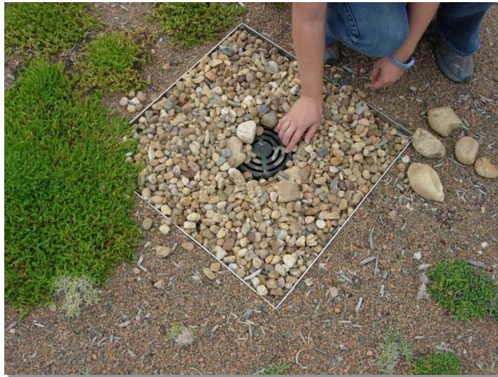
Photograph 6-3. When inspecting roof drains, remove any surrounding rock as well as the inlet grate and visually inspect the drainpipe to ensure it is free of any extraneous materials.
