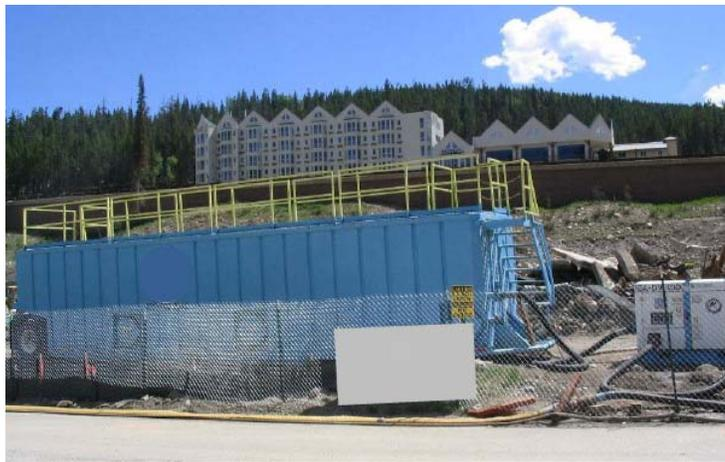
**Photograph CT-1.** Proprietary chemical treatment system being used on a construction site with sensitive receiving waters. Photo courtesy of WWE.
