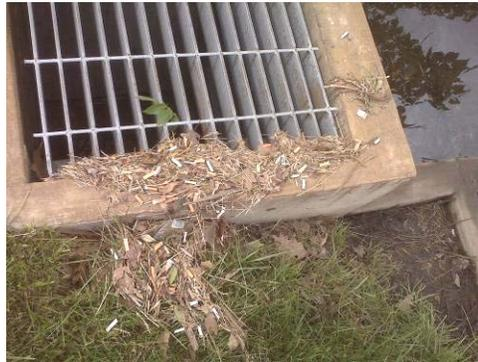
**Figure 14 Overflow of Light Particles in a PLDB**
