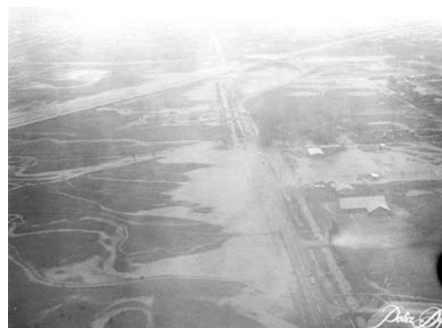
Looking west along South Boulder Road
