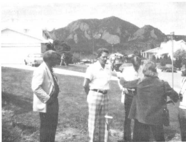
Boulder Mayor Penfield Tate, Boulder County Commissioner Wally Toevs and Boulder City Manager Archie Twitchell meet the press at Viele Channel groundbreaking.
