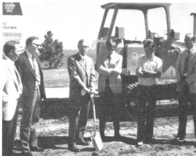
North Sanderson Gulch Groundbreaking — from left to right: Bud Rupert, Lakewood; Deryl Gingery, Gingery Associates, Inc.; Mayor James Richey, Lakewood; Scott Tucker, UDFCD; Dick Pascal, Pascal Construction Co.; Ray Bullock, Lakewood.
