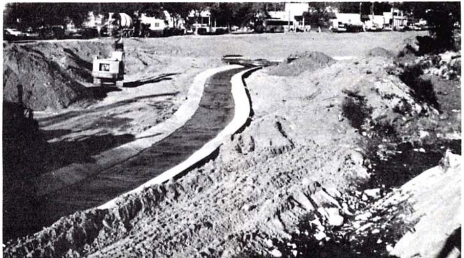
Lena Gulch at its confluence with Clear Creek in Wheat Ridge. This is another channel with a concrete bottom and rock sides.
