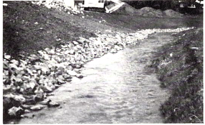
Figure 7 - Riprap used in a trickle channel.
