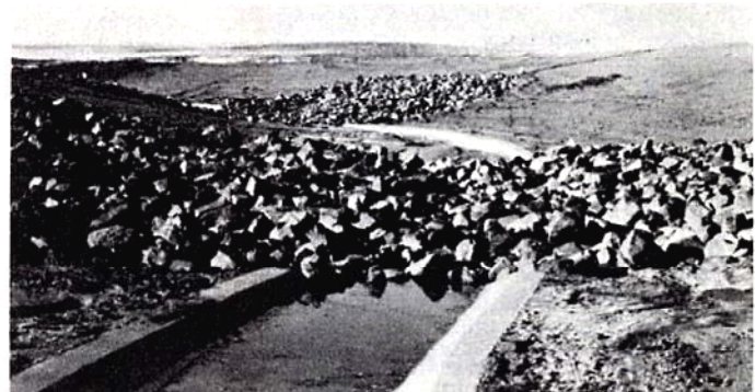
Figure 6 - Riprap can be used in drop structures.
