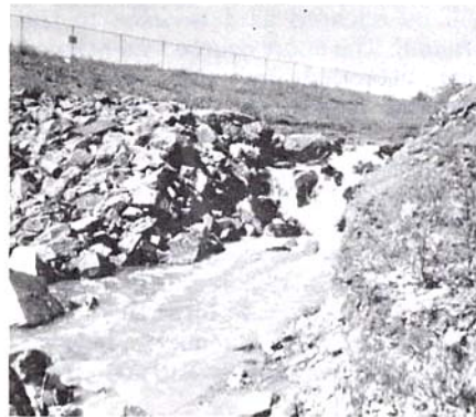
Figure 1 - Niver Creek Tributary L drop structure.
