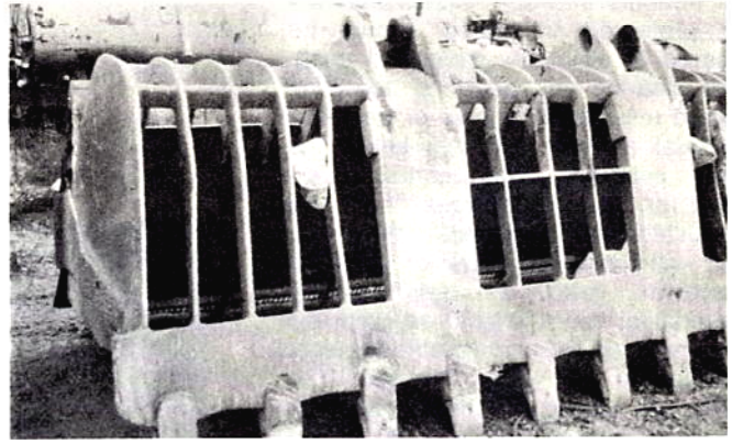
Figure 4 - A "rock bucket" which is used to sort out small rock pieces.
