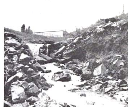
Figure 2 - Niver Creek Tributary L drop structure.
