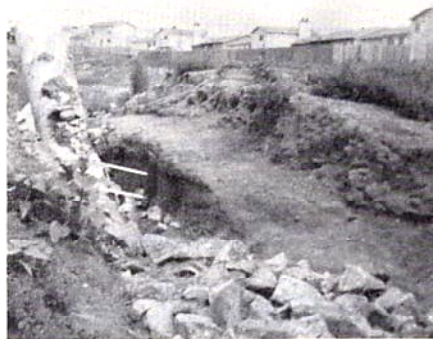
Figure 5 - Basin 0054 detention pond.
