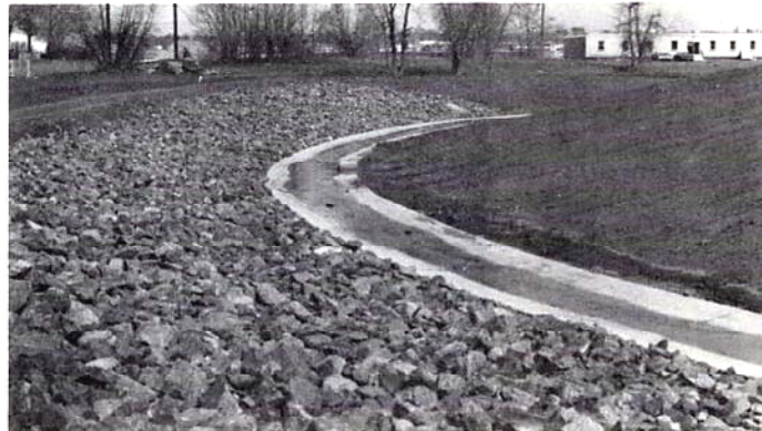
Figure 8 - Riprap used on a tight curve in a grass lined channel.
