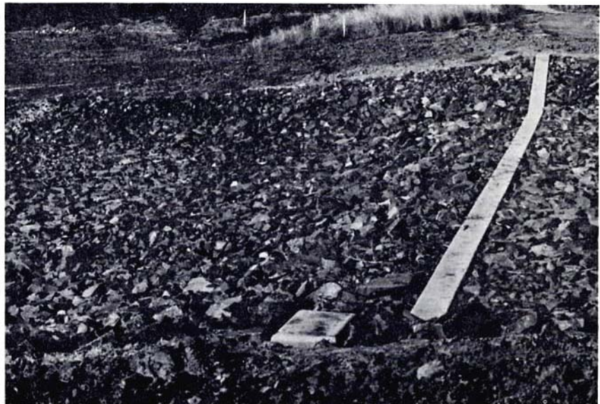
Riprap used to construct a spillway for a small detention pond.
