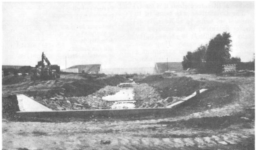
Westerly Creek Schedule IV looking upstream toward the Kelly Dam Spillway.
