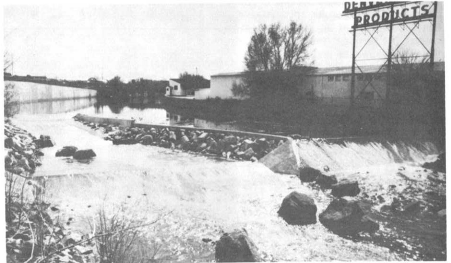
Photo 2 - Looking upstream at the Third Avenue Dam Bypass.
