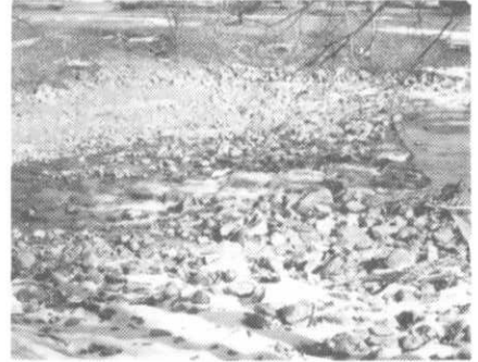
Cherry Creek drop structure.
