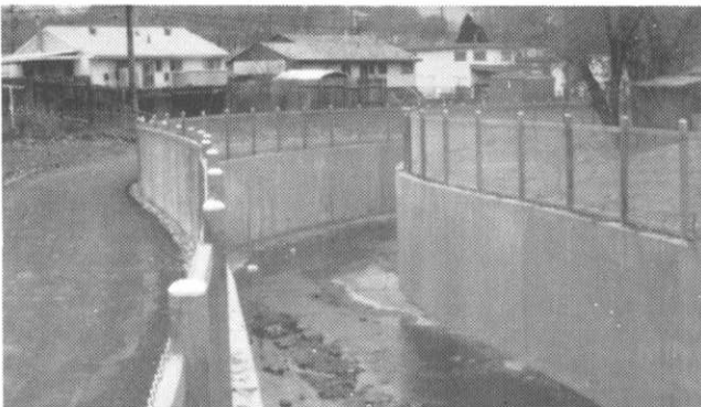
Weir Gulch Schedule 1 in Denver.
