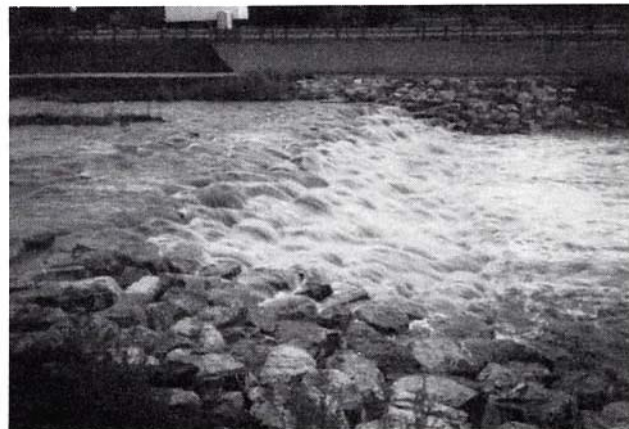
The finished structure during a minor flood event.
