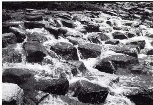
The finished structure at low flow conditions.
