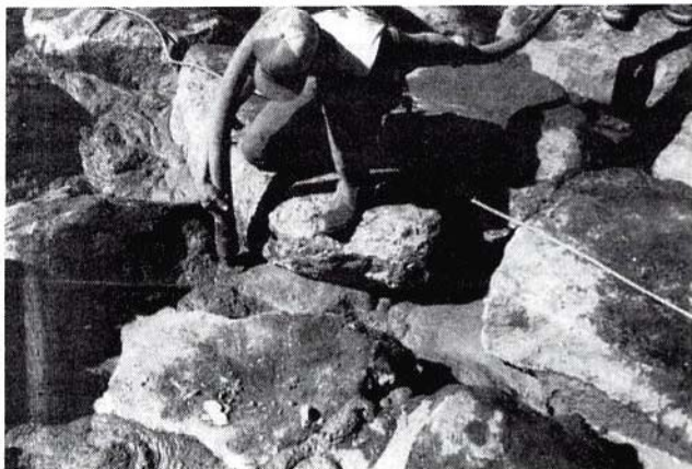
Placing the grout and vibrating it into place.
