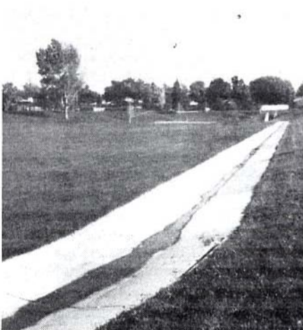
The recently completed Rotary Park Detention Pond.
