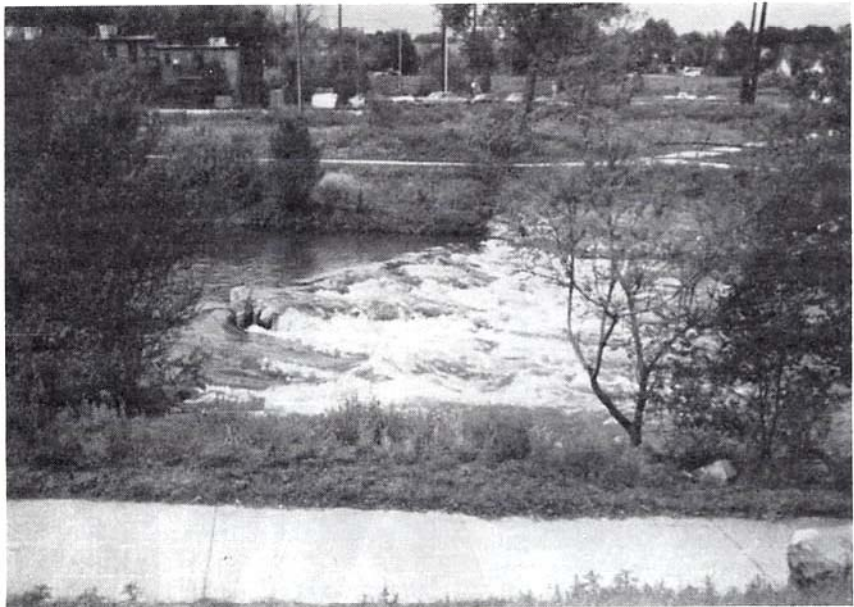
The new grade control structure at 19th Street. Note the boat passage at the right side of the structure.
