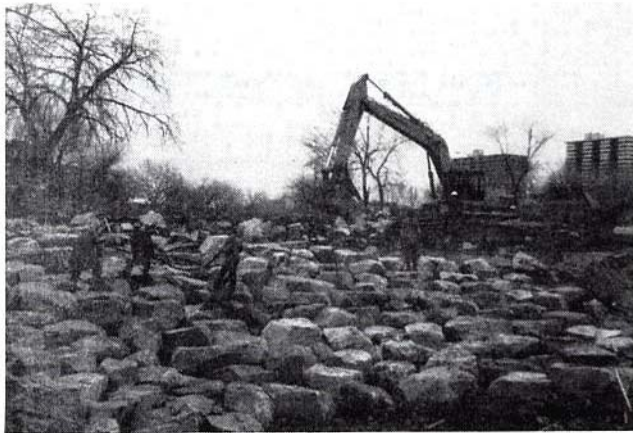
Setting the boulders in place using a back hoe.
