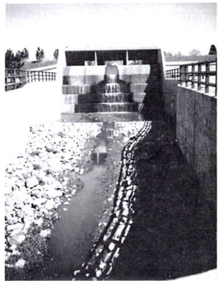
Looking upstream at the Little's Creek crossing of the railroad depression.
