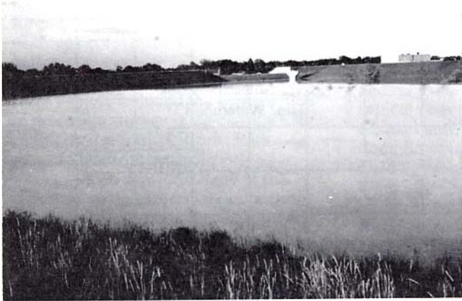
Kelly Road Dam, normally dry, on Westerly Creek on June 6, 1991.
