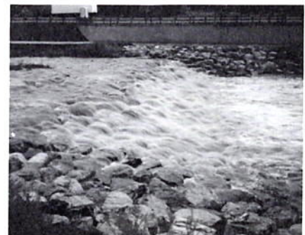
One of the grouted sloping boulder drop structures in Cherry Creek Park.
