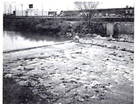
Before and after views of the Mississippi Ave. check structure.
