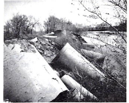
Debris at the Eppinger property prior to beginning the cleanup.
