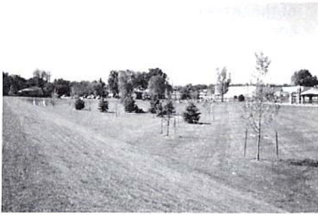
The recently completed Citizens Park Detention Pond in Edgewater.
