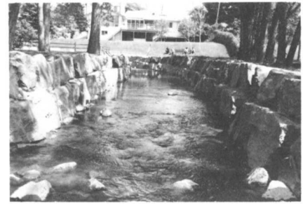
Dry Gulch boulder lined low flow channel.
