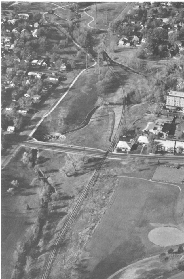
Circular drop structure on Dry Gulch (center left) and confluence of Lakewood Gulch and Dry Gulch (top center), a joint flood control and recreation project.
