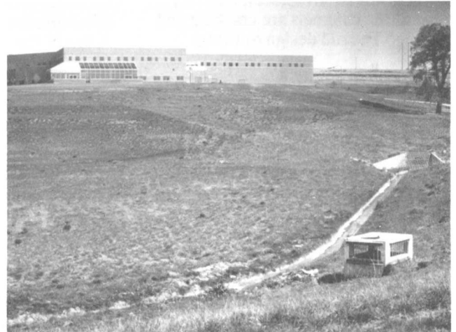
Figure 5. Pond "D" in Louisville taken from the embankment. The outlet works is in the foreground and the new recreation center is in the background.
