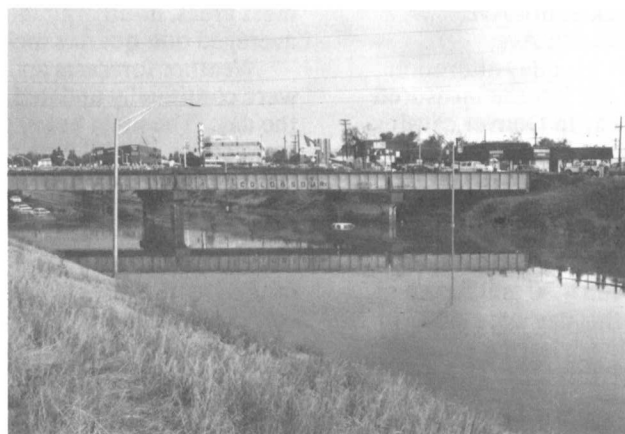
Figure 3. I-25 at Evans Ave. on July 20, 1992.
