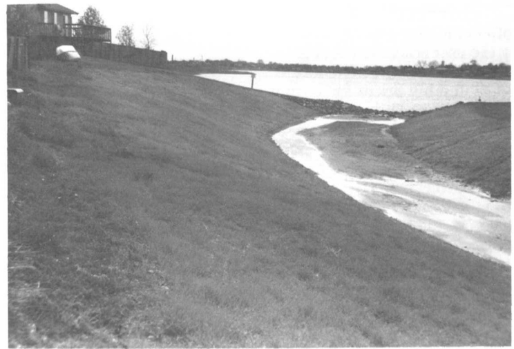
Before and after views of the Hidden Lake inlet channel maintenance.
