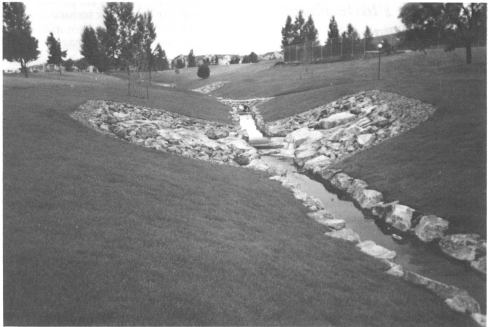
Four Lakes Tributary channel in Arapahoe County.
