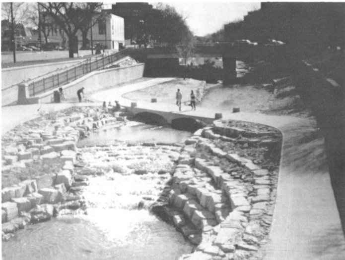
One of the Creekfront drop structures.
