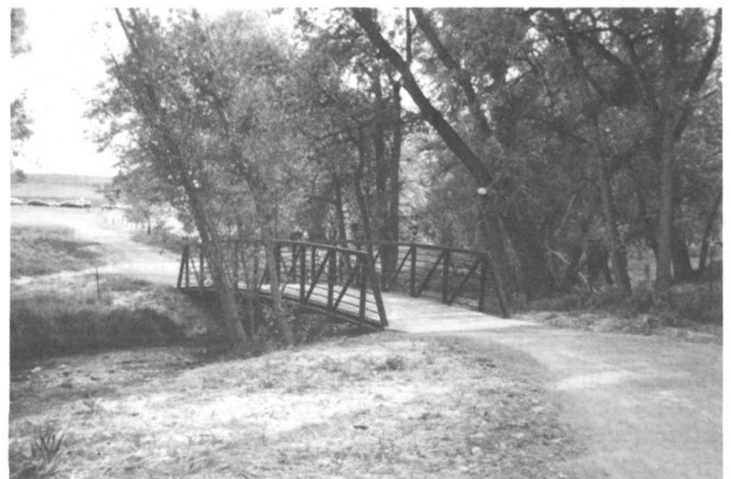
Maintenance access/recreation trail on Coal Creek in Lafayette.
