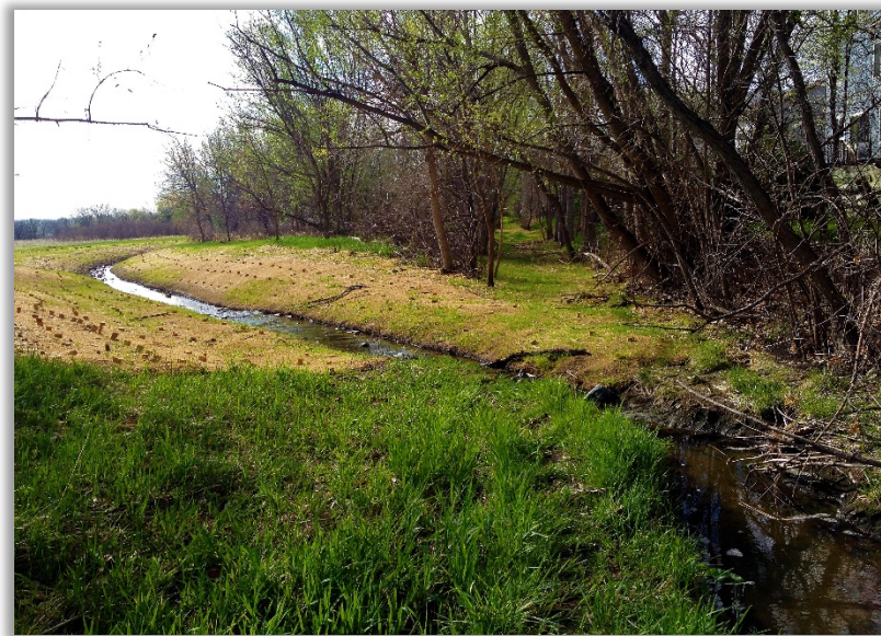
Nissen Reservoir Drainageway
