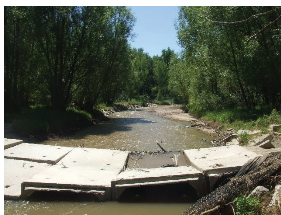
Figure 5: Plum Creek Main Channel Braided with Sandy Bottom ( 0.025 < n < 0.030 )
