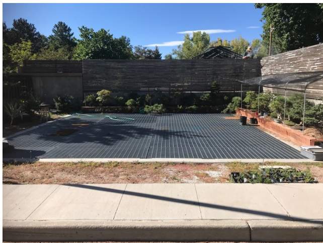
Photograph SF-2. Underground sand filter at Denver Botanic Gardens has a grated top, which enables inspection and maintenance.
