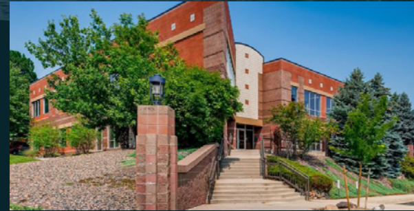
Our new location at 12575 W Bayaud Ave in Lakewood
