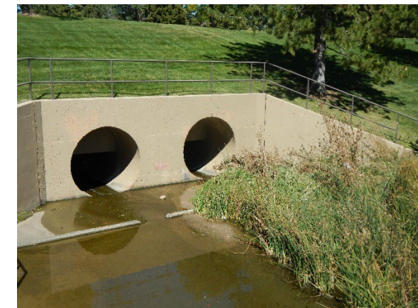
Basin outlet looking north.
