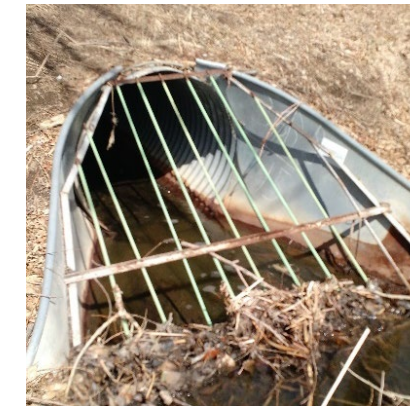
Basin outlet looking north.
