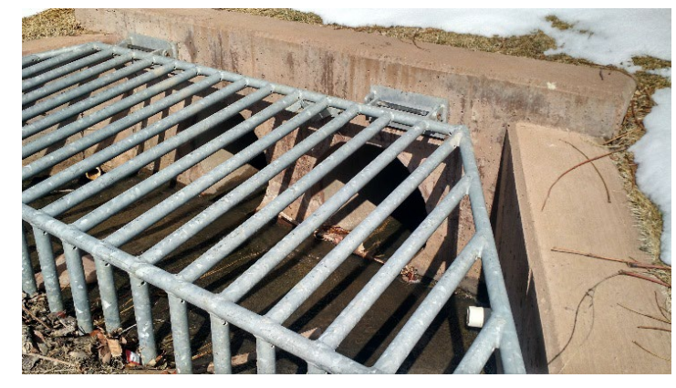
Basin outlet looking north.
