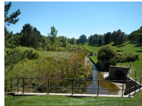
Basin looking south from the outlet.
