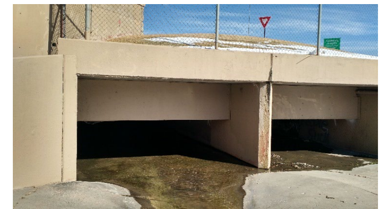
Basin outlet looking north.
