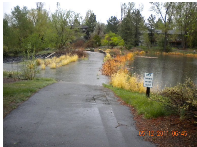
Orchard Hills detention spillway looking east.
