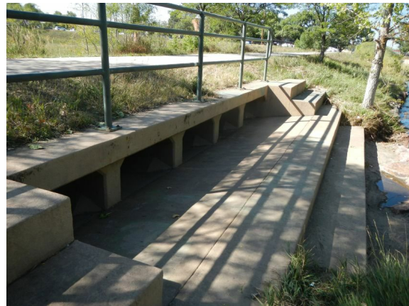
Basin inlet looking northwest.
