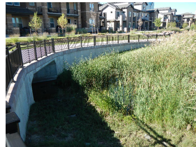
Basin inlet looking south.
