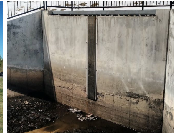
Basin outlet looking north.
