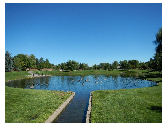
Basin and inlet looking north.
