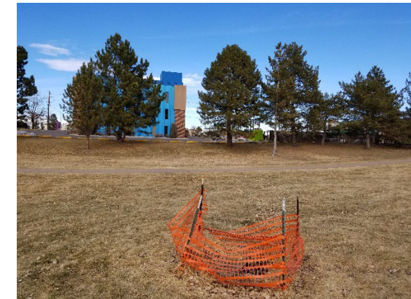
Basin outlet and spillway looking north.
