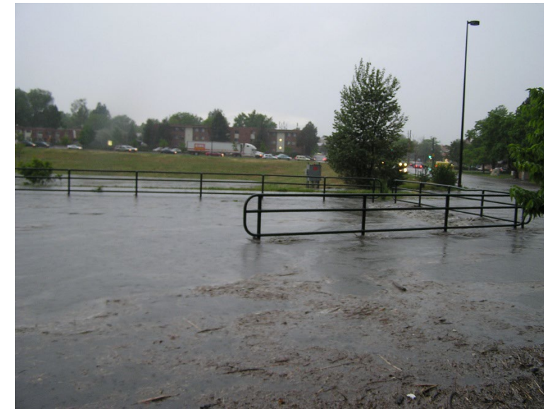
Goldsmith Gulch at Iliff Avenue looking west along Iliff Avenue towards the detention basin.
