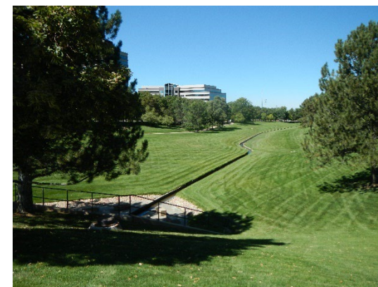
Basin inlet looking north.
