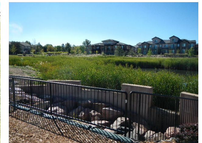
Basin outlet looking south.
