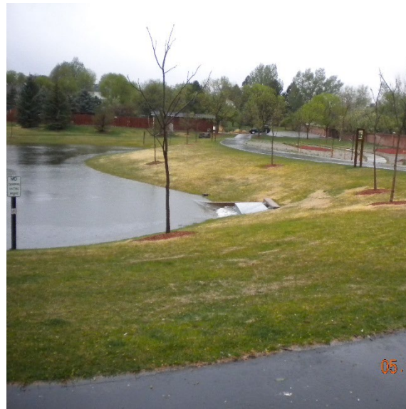
Tommy Davis Park detention outlet (on south side of berm) looking west.
