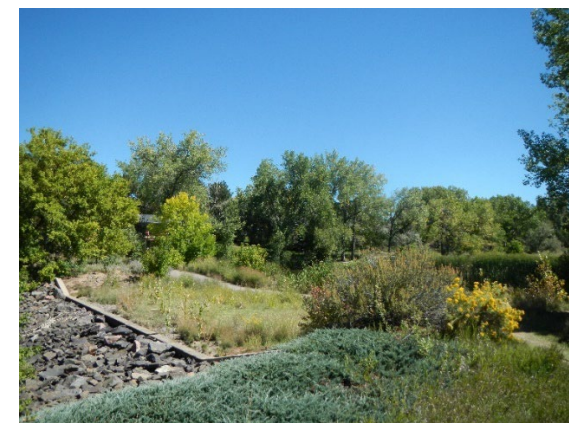
Basin spillway looking east.
