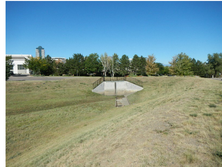
Basin and outlet looking north.
