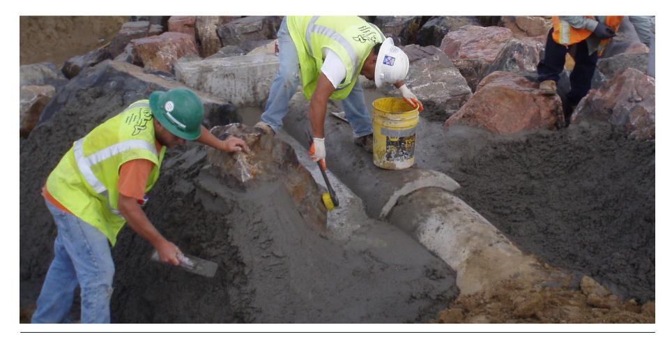
**STEP 9 (Curing):** After grout is placed and the boulders are cleaned, the grout shall be cured. Confirm that appropriate curing methods and hot/cold weather protection are implemented:
