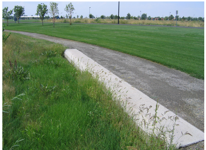
Photograph 4-12. Aurora Sports Park Level Spreader. This level spreader carries concentrated flows into a slotted pipe encased in concrete to distribute flows evenly to the RPA shown left in the photo. Photo: Wenk.
