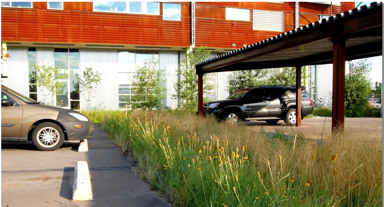
Photograph 3-3. Unconnected impervious area (UIA) draining to receiving pervious area (RPA). Vegetated buffer strips and/or raingardens are common ways to disconnect impervious area in parking lots.
