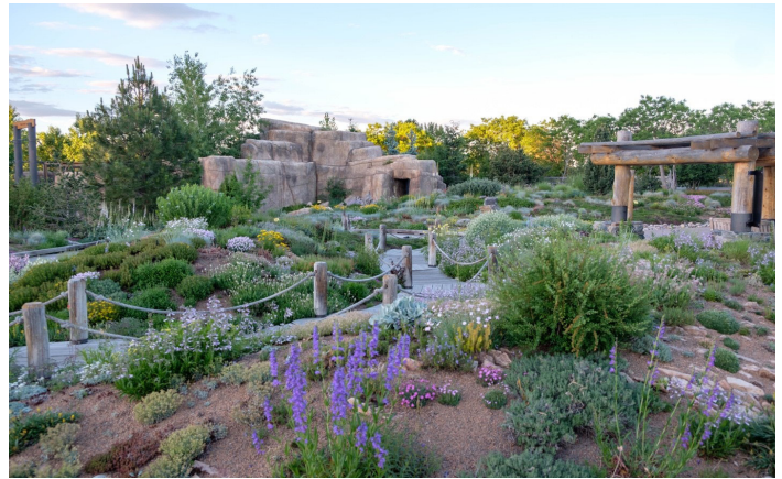
Photograph GR-2. Denver Botanic Gardens intensive green roof over parking garage. Photo: Michael Guidi.
