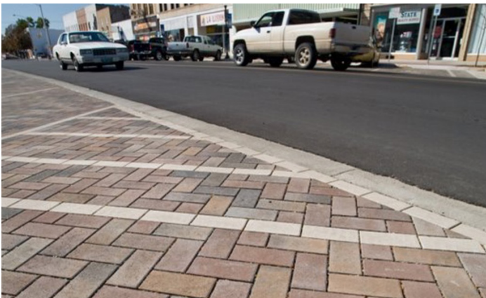
Photograph PPS-3. PICP in downtown Ft. Morgan, CO. Note soldier course of light-colored pavers where PICP meets conventional pavement. Photo: SEH and the City of Ft. Morgan.
