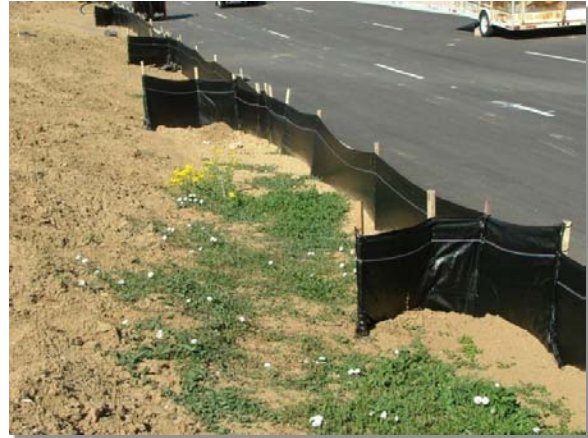
Photograph SF-2. When silt fence is not installed along the contour, a "J-hook" installation may be appropriate to ensure that the BMP does not create concentrated flow parallel to the silt fence. Photo courtesy of Tom Gore.
