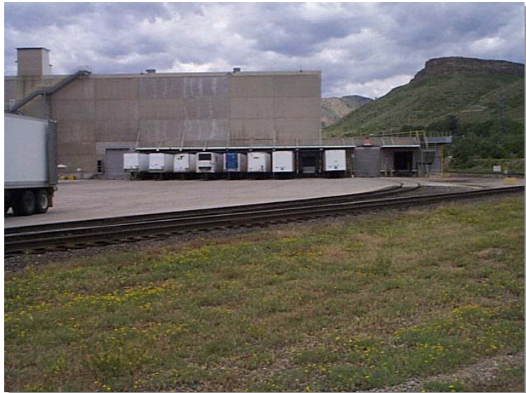
Photograph CS-1. Covered truck loading dock helps reduce exposure of materials to runoff.
