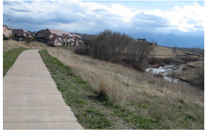
Photograph RPA-4. Grass buffers can be used to manage runoff from parking lots, multi-use paths, roadways, or roof areas, provided the flow is distributed in a uniform manner over the width of the buffer. Native grasses provide a more natural appearance. Photo: WWE.
