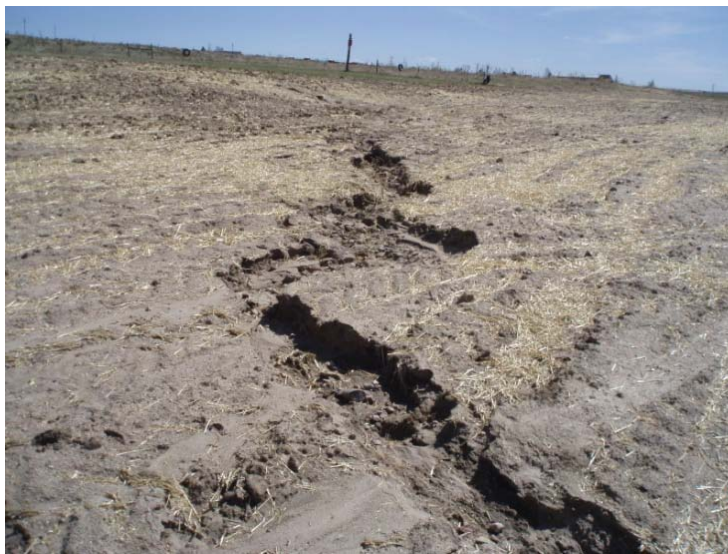
Photograph 7-2. Diverting the upland slope drainage area may have avoided the rilling shown in this picture.
