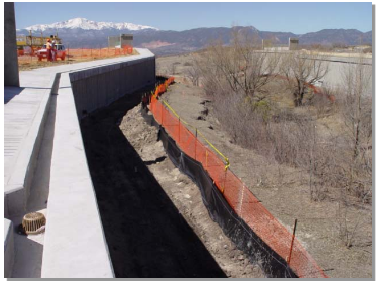
Photograph PV-1. Protection of existing vegetation and a sensitive area. Photo courtesy of CDOT.
