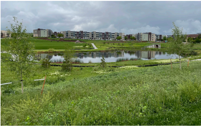
Photograph RP/CWP-1. Retention ponds and constructed wetland ponds treat stormwater through sedimentation and biological processes including uptake.
