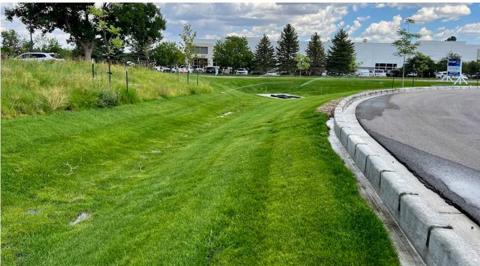
Photograph RPA-2. RPAs including grass buffers and swales treat runoff by filtering and infiltration. For treatment to be effective, grass buffers must receive runoff as sheet flow. Photo: WWE.
