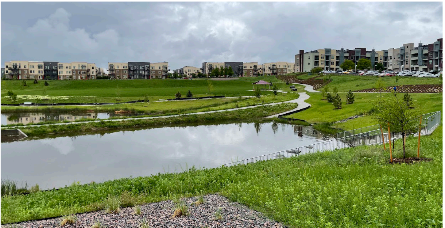
Photograph RP/CWP-3. Variations in slope and texture around the pond, trails, and pavilions connect this retention pond to the community as a recreational and aesthetic amenity.
