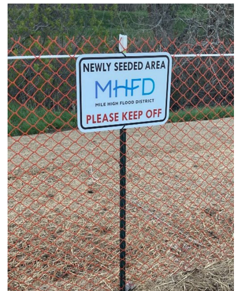
Photograph RPA-11. Signage and construction fencing can help protect the RPA as vegetation becomes established.
