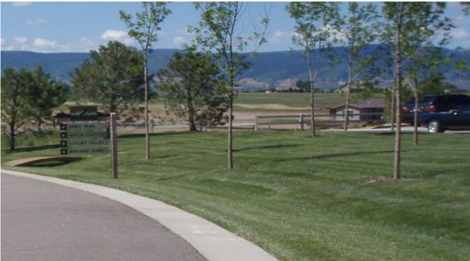
Photograph RPA-1. Grass buffers are often used in conjunction with grass swales as a treatment train. These pervious areas also help reduce heat island effects in urban areas. Photo: Muller Engineering.
