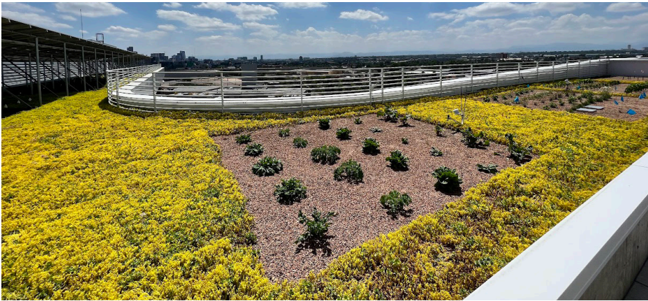
Photograph GR-3. Intensive green roof over parking garage is readily accessible for maintenance.
