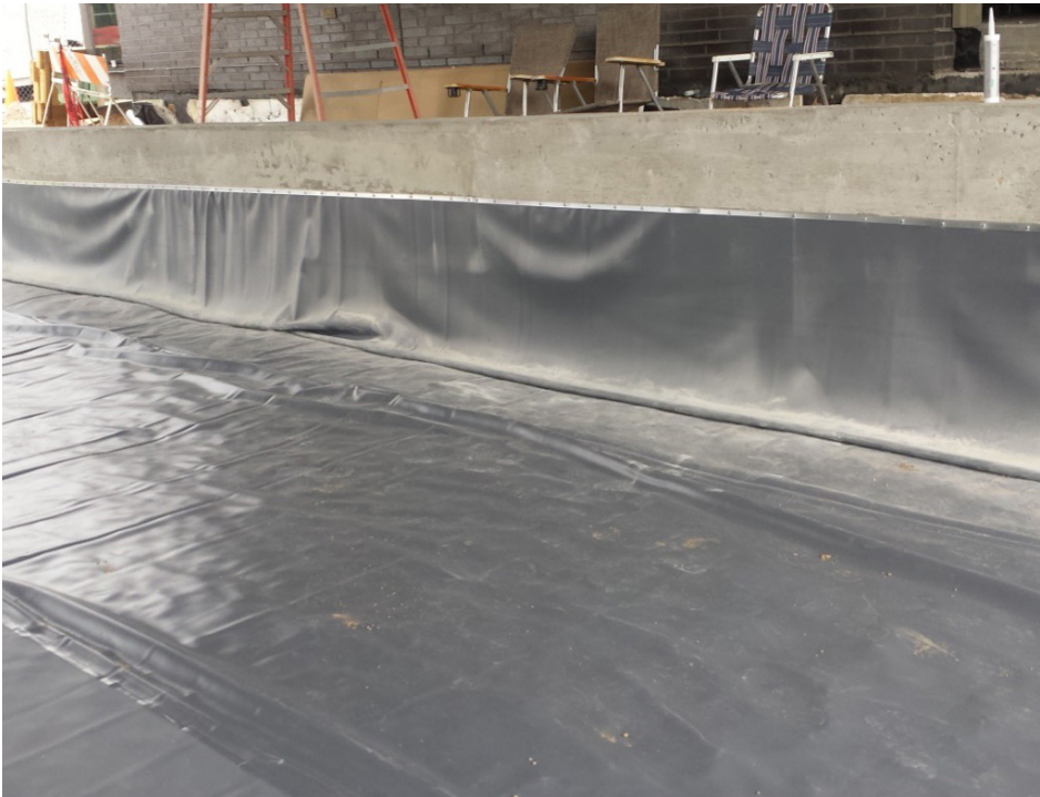
Photograph PPS-10. Geomembrane attached to concrete perimeter barrier. Photo: Creative Civil.
