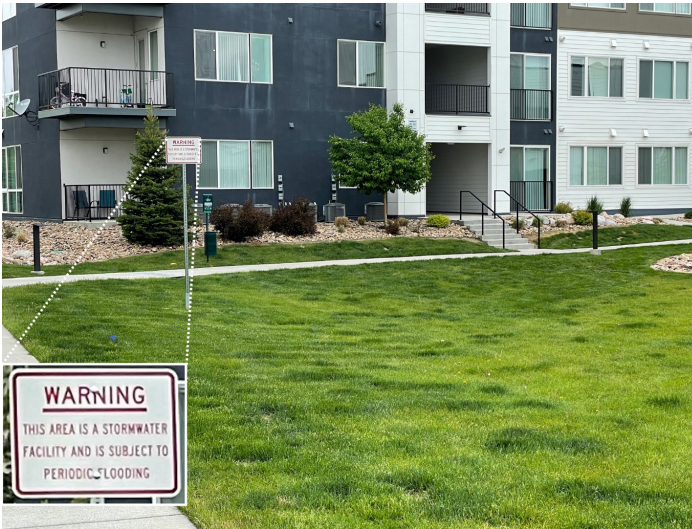
Photograph RPA-7. RPA in multi-family residential neighborhood. Sign warns of periodic flooding which helps establish expectations for periodic temporary ponding, while providing a safety warning. Photo: WWE.
