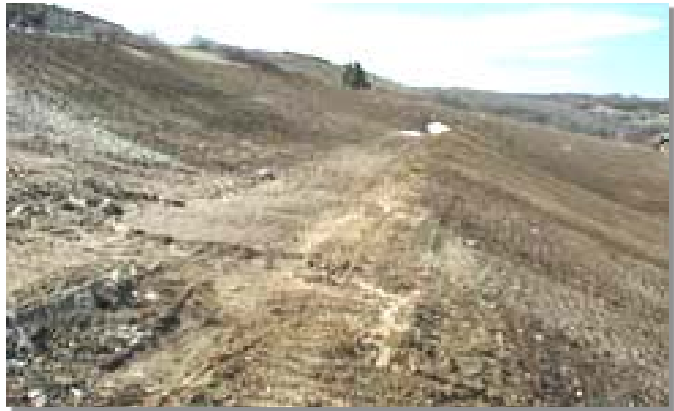
Photograph TER-1. Use of a terrace to reduce erosion by controlling slope length on a long, steep slope. Photo courtesy of Douglas County.
