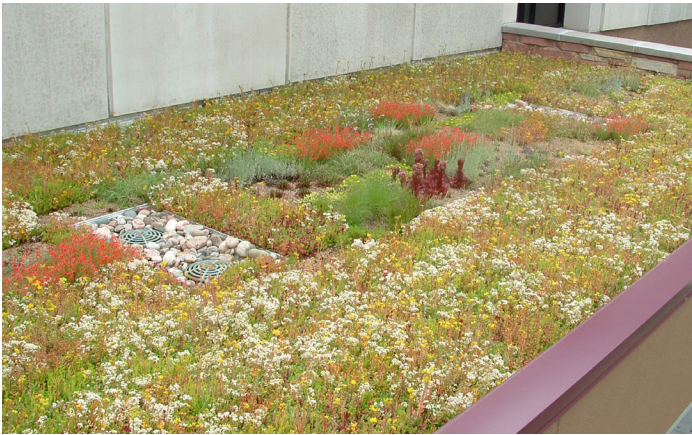
Photograph GR-1. Extensive Green Roof. Photo: Jennifer Boussetot.
