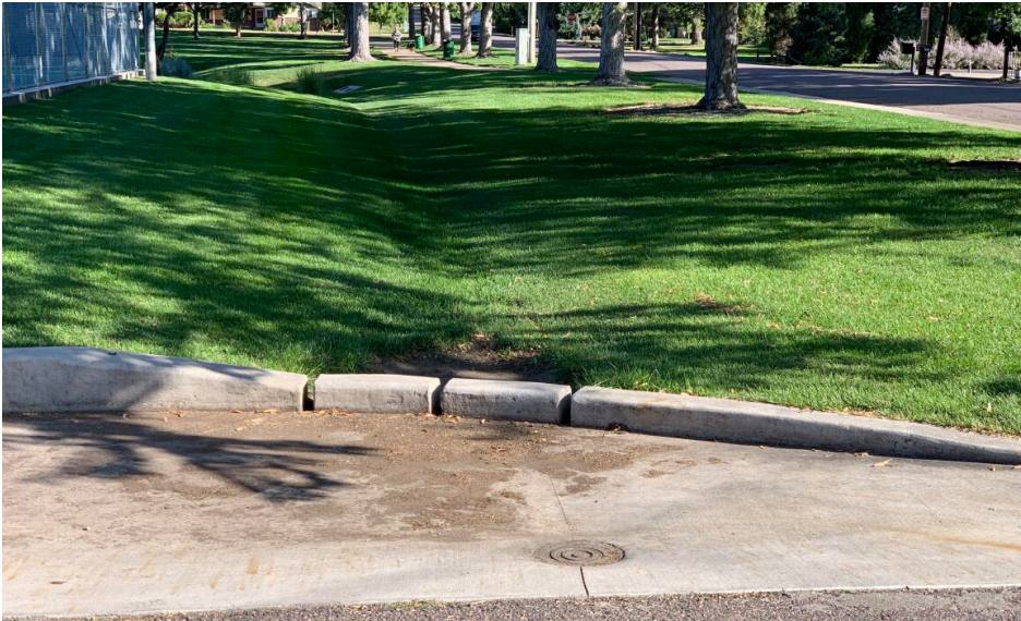
Photograph RPA-10. Sediment forebay at the entrance to a grass swale leading to an EDB concentrates maintenance needs at entrance of swale. This is an example of a three-step treatment train: forebay, swale, pond.
