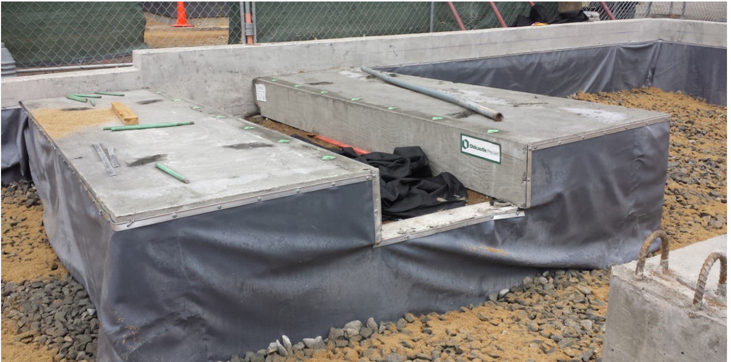
Photograph PPS-12. Tree planter vault for PICP installation. Photo: Creative Civil.
