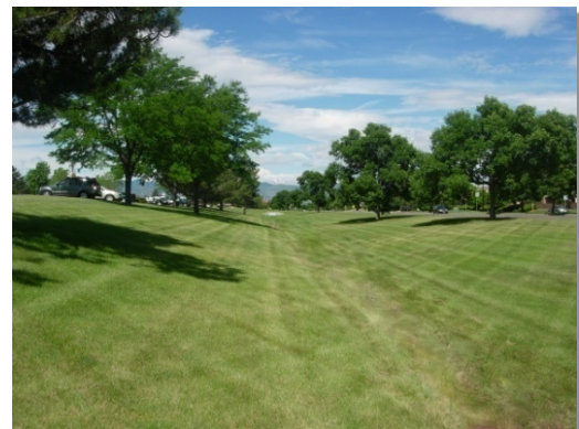
Photograph 1-3. Grass Swale. This densely vegetated grass swale is designed with channel geometry that forces the flow to be slow and shallow, facilitating sedimentation while limiting erosion.
