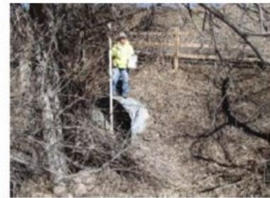
Reach WC-5: Structure 17 – Bellevue Avenue (1) 72-inch CMP
