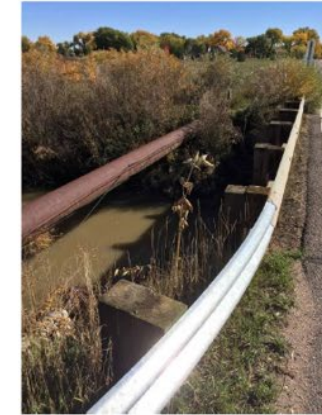
Figure 9-11: Kenosha Rd Bridge Downstream
