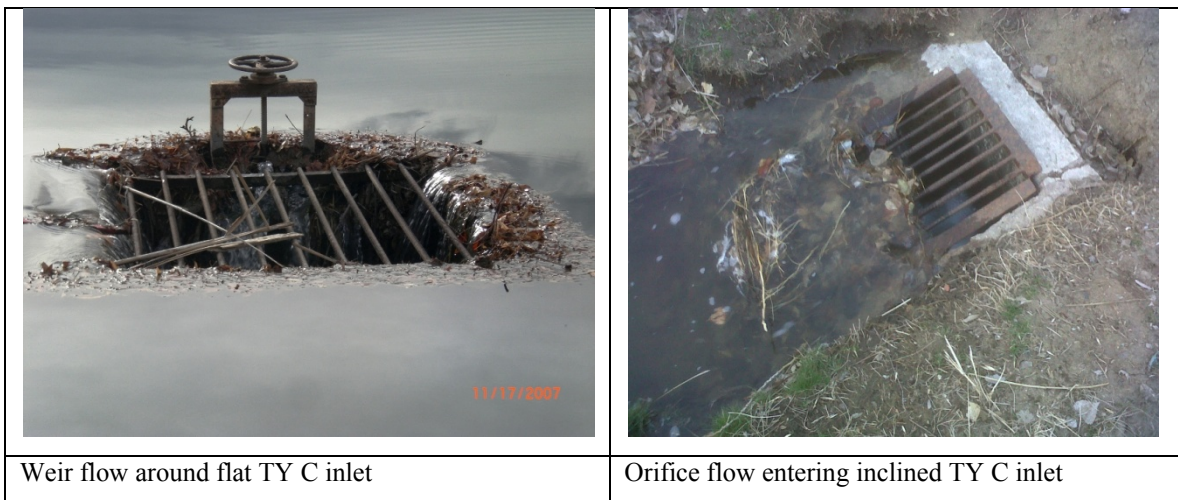
Figure 3 Flow Hydraulics around Type C Inlet
